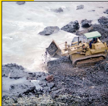
Surfwashing: Pushing polluted sediment down the beach in the surf zone (mid-tide) Recover the released oil (nets)
