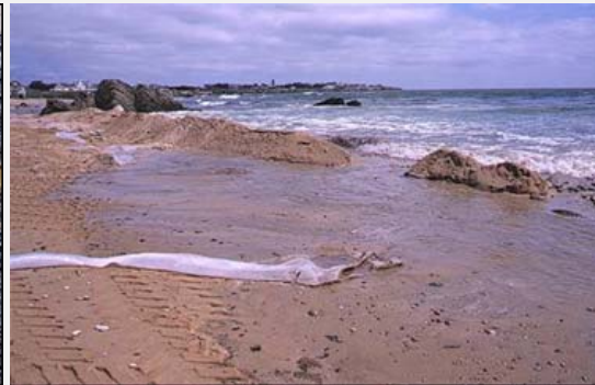
Surfwashing: Pushing polluted sediment down the beach in the surf zone (mid-tide) Recover the released oil (nets)
