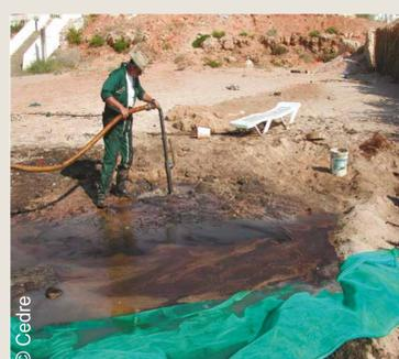
Water agitation of sediment with low pressure jet
